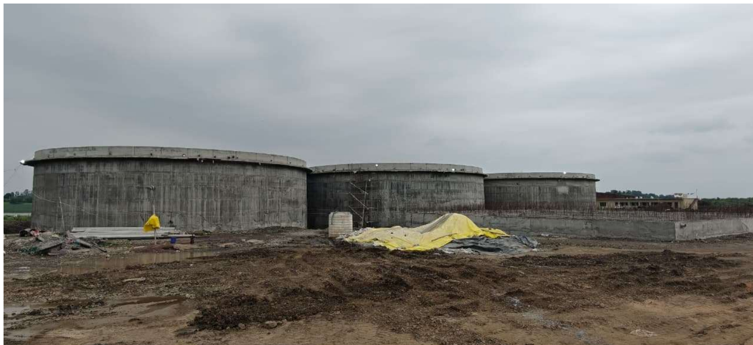
CBG Organics' plant under construction in Guna.
